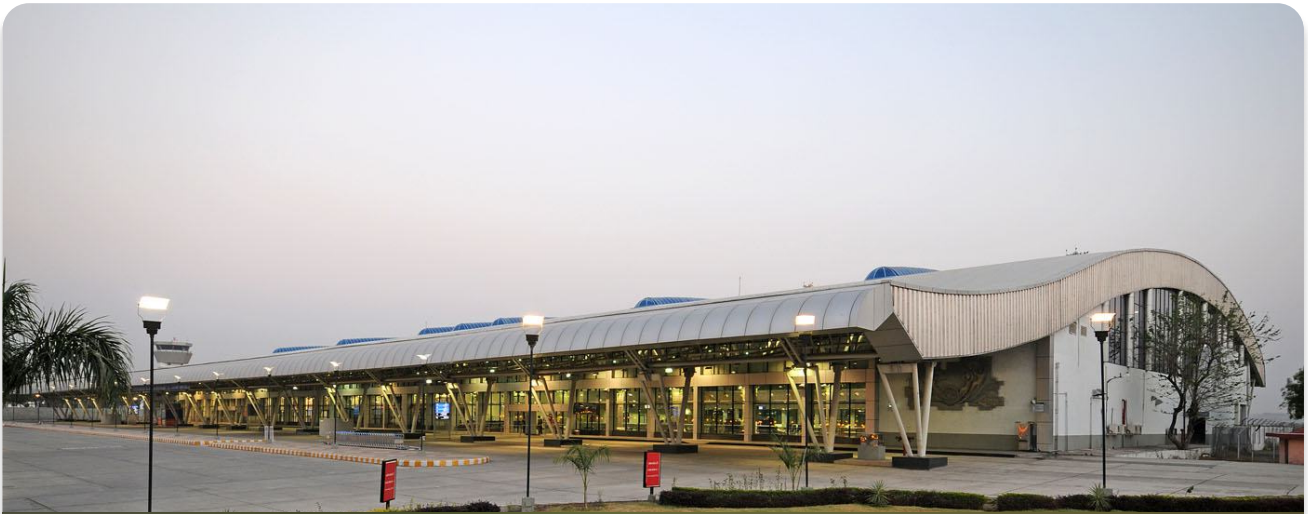
Raja Bhoj International Airport Bhopal, Madhya Pradesh
